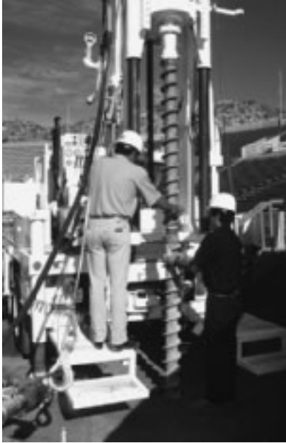
Figure 18.2 Drilling with flight augers (Courtesy of Danny R. Anderson, PE, of Professional Service Industries, Inc., El Paso, Texas)
