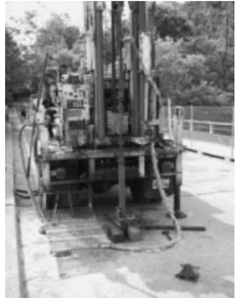
Figure 18.7 Drilling rod with split-spoon sampler lowered to the bottom of the borehole (Courtesy of Braja M. Das, Henderson, Nevada)
